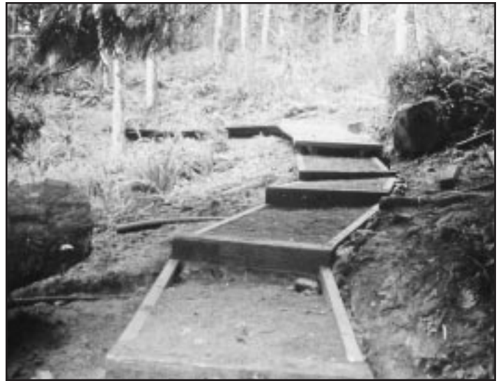
Stair risers at puncheon.
