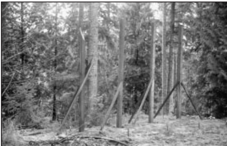
Kiosk under construction at uneven aged management area.
